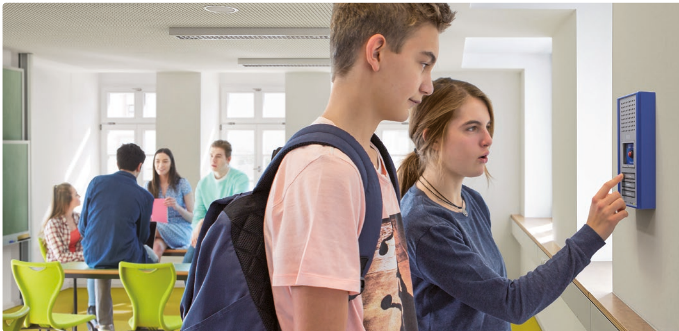
Intercom systems make it possible to communicate with the permanently occupied post and receive instructions in the event of an emergency.
