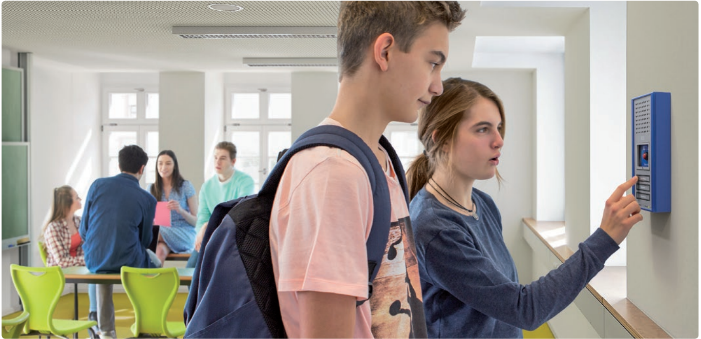
Intercom systems make it possible to communicate with the permanently occupied post and receive instructions in the event of an emergency.
